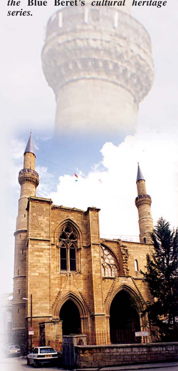
The front entrance
