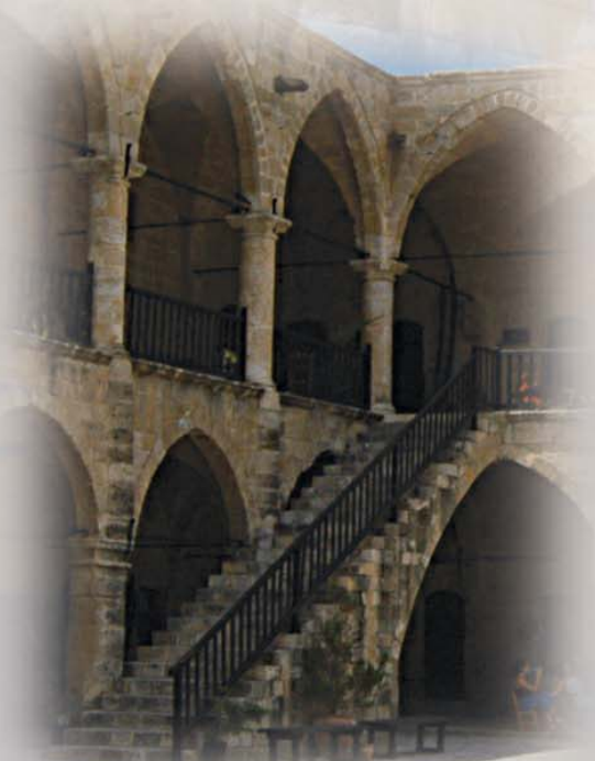
Staircase leading to the upper floor
