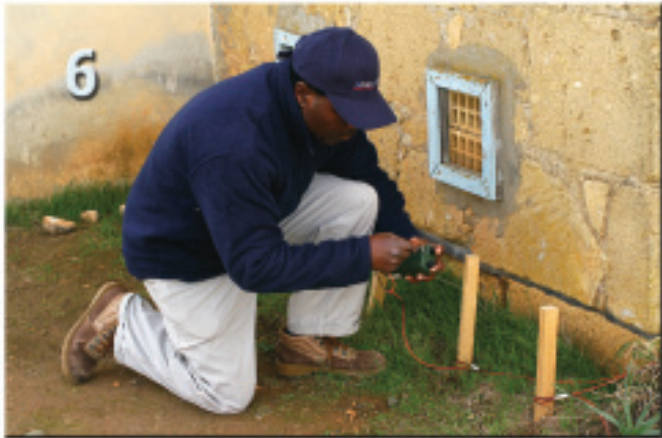
Connecting Firing Circuit
